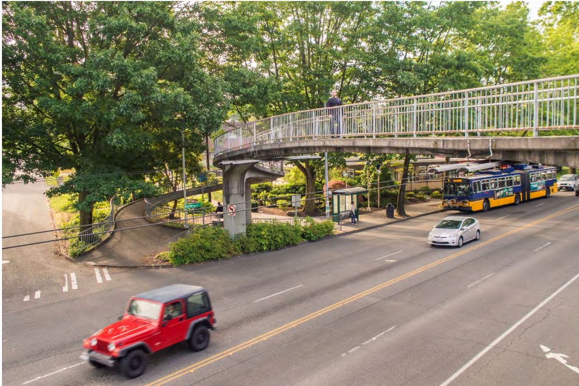
Pedestrian bridge at Mount Baker, Seattle, Washington
