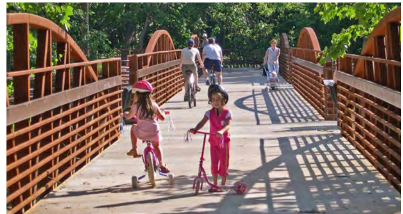
Bicycle & Pedestrian Bridge Source: Public Square, 2018
