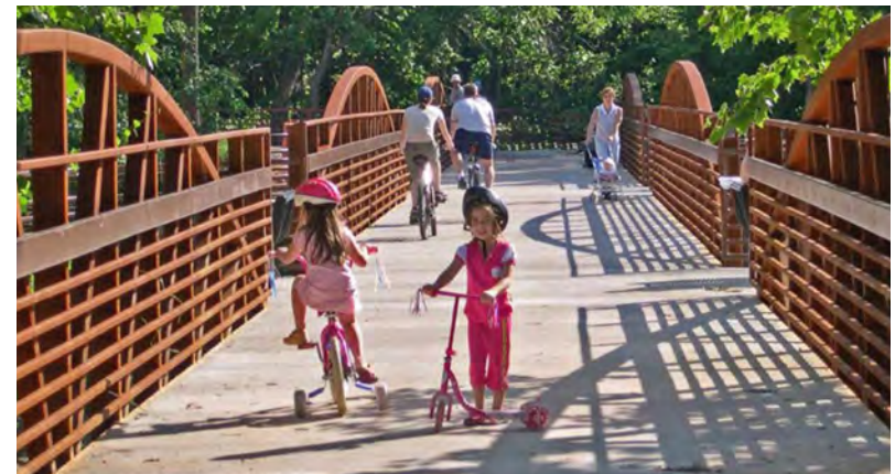
Bicycle & Pedestrian Bridge Source: Public Square, 2018
