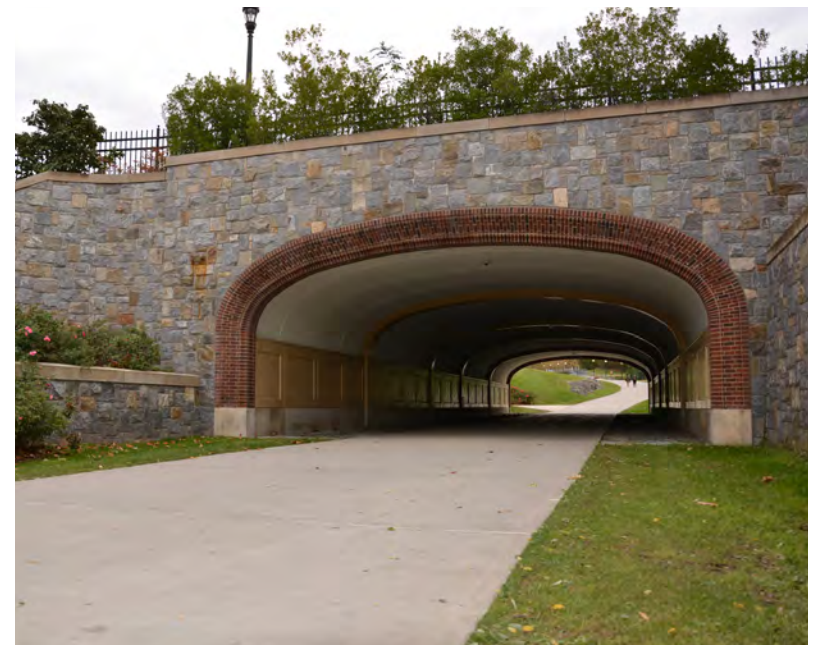
Example of Pedestrian Undercrossing Source: Schultz Heavy Civil Construction, 2020
