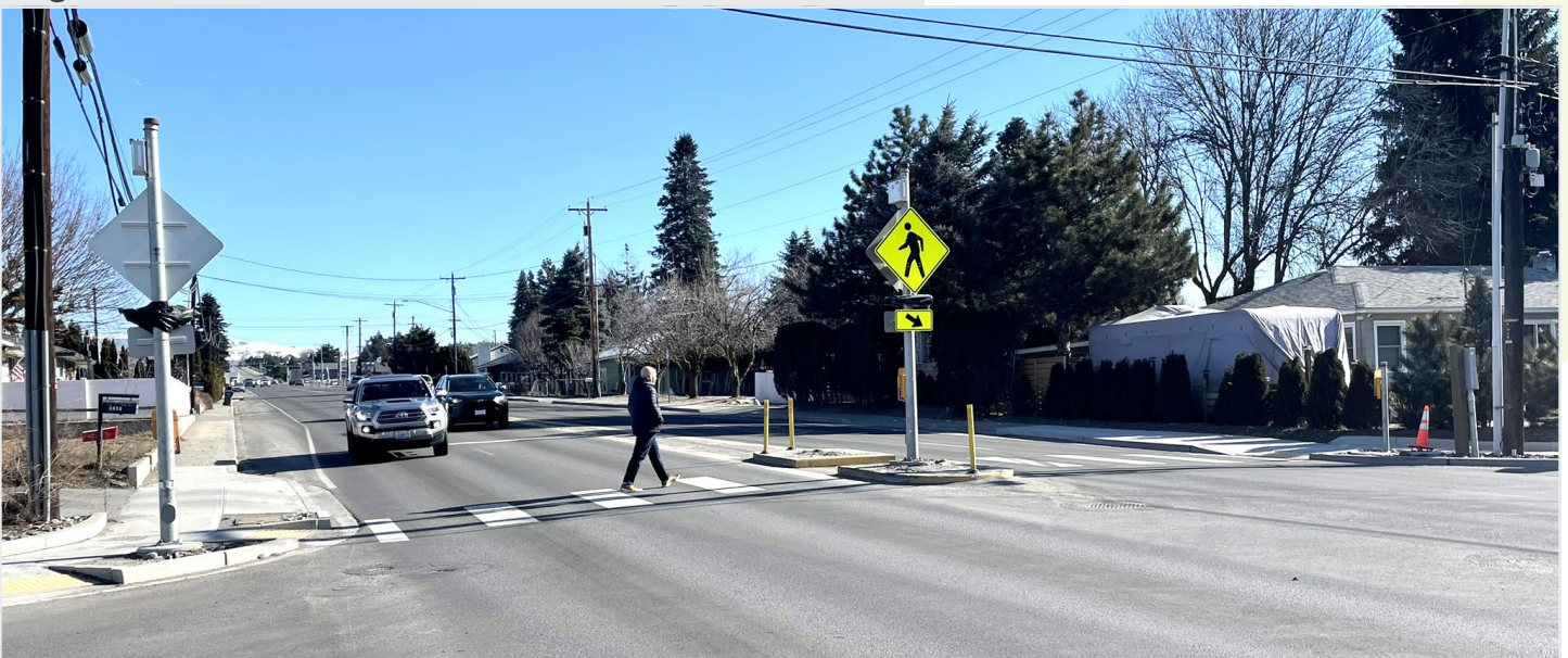
Figure 2-3: Suburban Road in East Wenatchee
