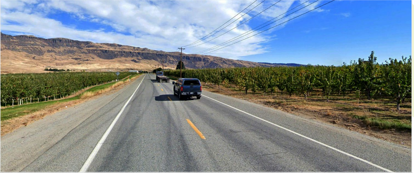
Figure 2-2: Rural Road in Douglas County
